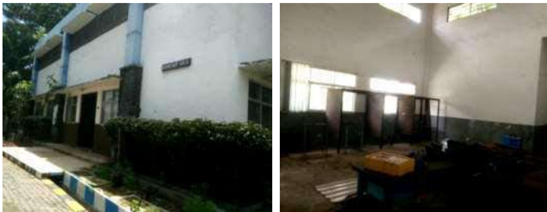
Gambar 5.8 Workshop Kerja Baja
