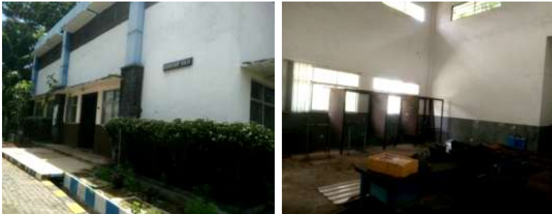
Gambar 5. 8 Workshop Kerja Baja
